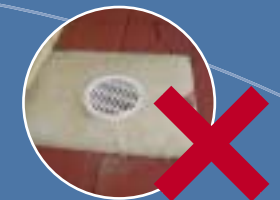
In both of these cases the paving and landscaping is too high - stormwater will flow into the ORG, potentially causing a sewage overflow.
